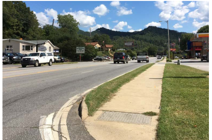
Figure 4: Pedestrian/bicycling facilities along NC 107
