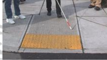
Fig. 4-1: Truncated domes help the visually impaired determine where the sidewalk meets the street.
