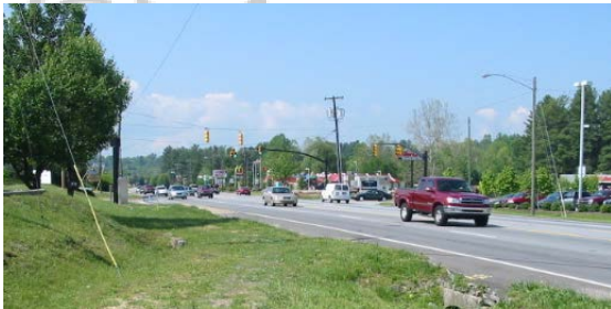
Fig. 2-2: This section of sidewalk on Broad Street near Chestnut Street (seen left of center in this photo) leaves pedestrians with no refuge from swift-moving traffic.
