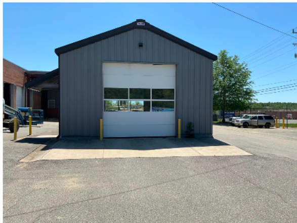
Construction around structure
